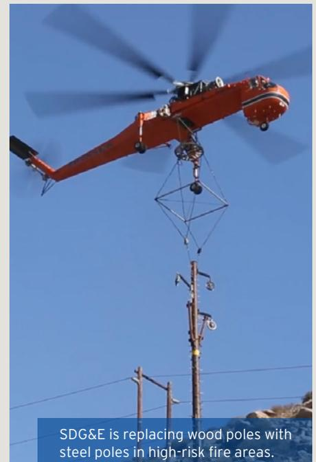
SDG&E is replacing wood poles with steel poles in high-risk fire areas.
