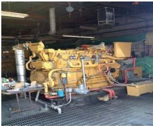
The objective of this demonstration was to identify a reliable, cost effective method to achieve SCAQMD Rule 1110.2 compliance using digester gas (DG) fuel for engines. In 2015, Tecogen emission control technology was successfully installed on a rich burn engine that runs on digester gas at the Eastern Municipal Water District water treatment facility in Perris, California. The engine and emission control system successfully ran throughout 2016. This project has been completed.
