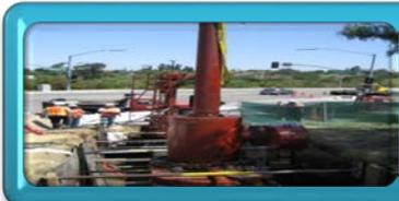
Isolate Small Section Using Stopples-infrequently
